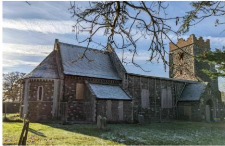
North Side of Church from Sanctuary Side
