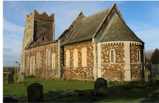
South Side of Church from Sanctuary Side.
