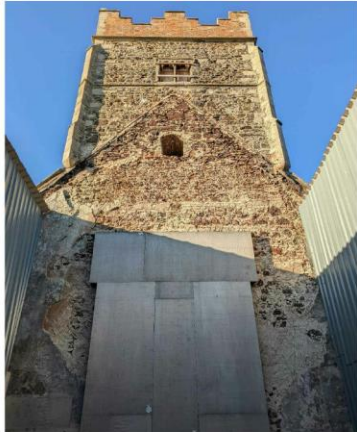
Looking Towards the Tower from Nave
