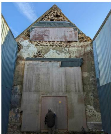
Looking at Chancel Wall from Nave
