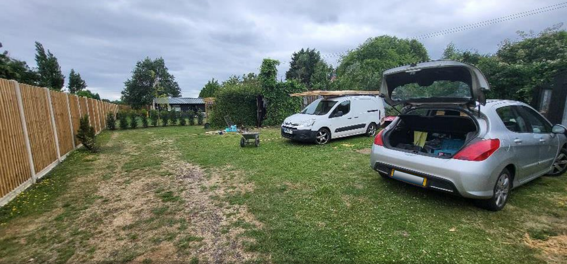
Parking area in rear garden of dwelling, kennel building in background
