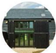
Sliding 'Barn' Doors
