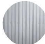
Profiled metal roof
