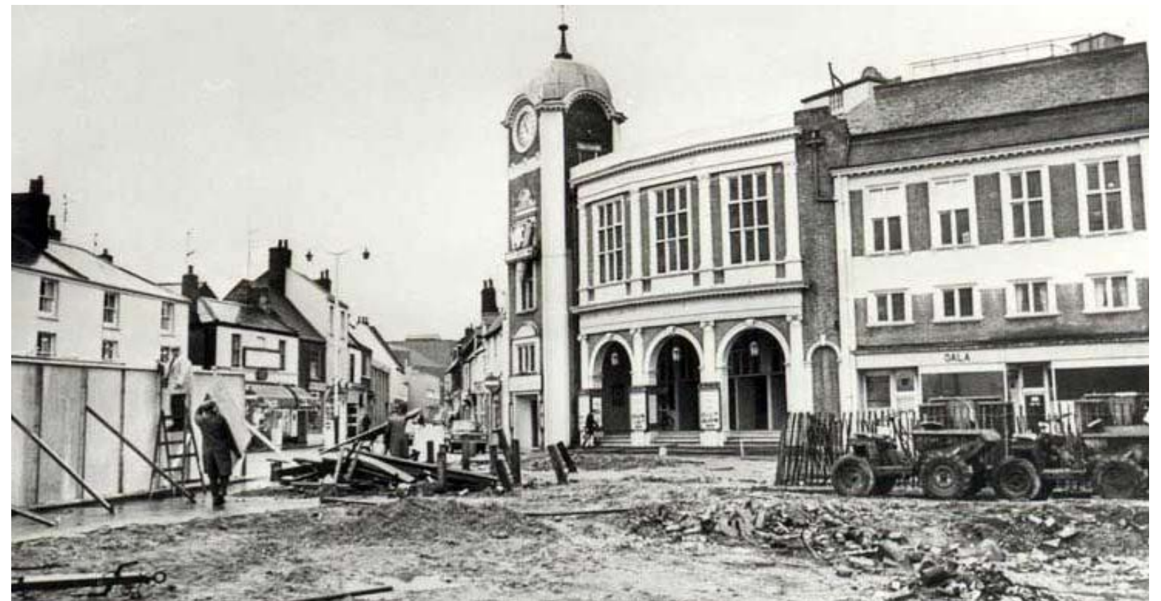
Historical Photograph of the site prior to construction of the existing building
