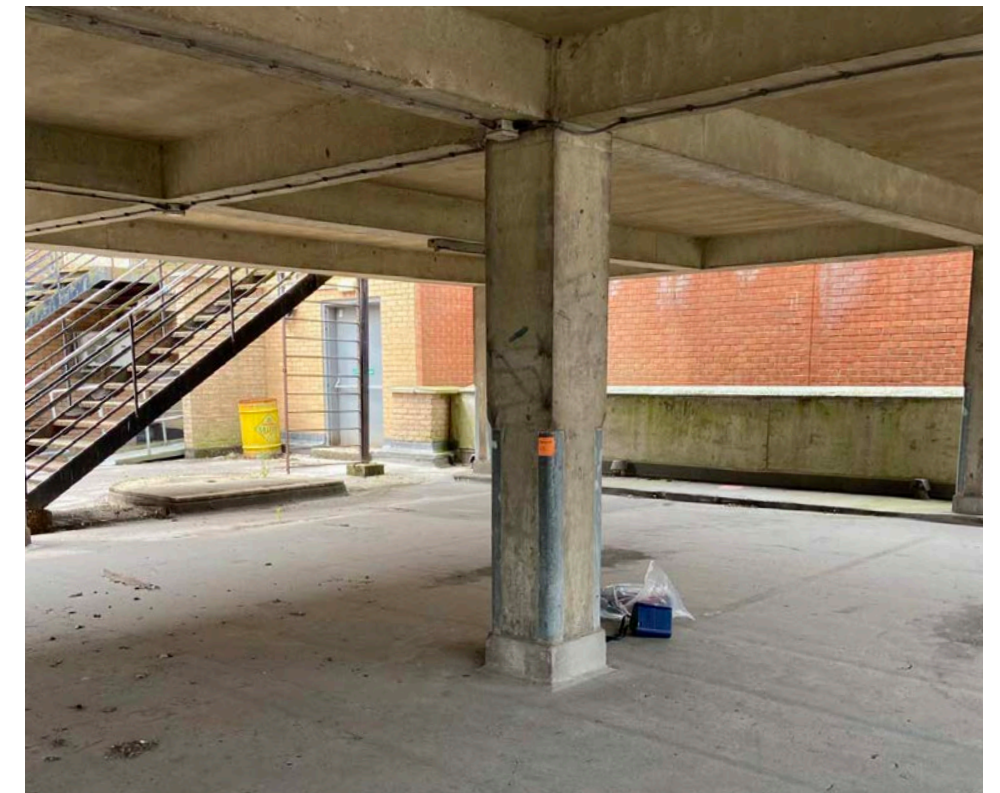
Existing second floor - exposed structural frame
