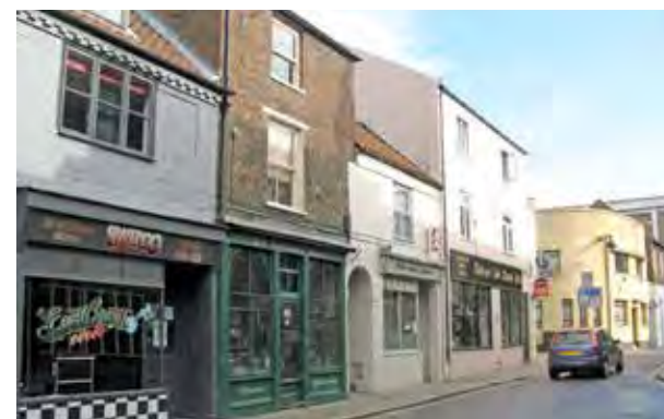
St James' Street west end
