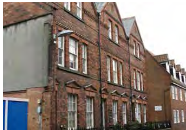
Nos. 22, 24 and 26 Queen Street
