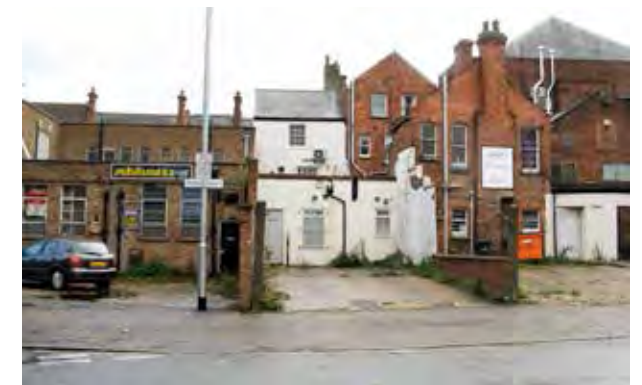
Back boundaries to the shops in the High Street from the Baker Lane car park
