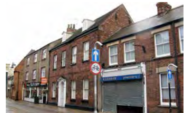
Whincop House, Tower Street
