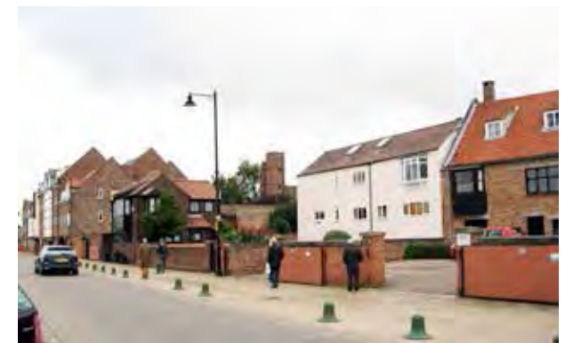
South Quay showing view to lookout tower of Clifton House
