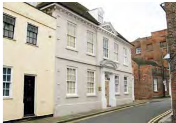
No. 19 Nelson Street (Oxley House)
