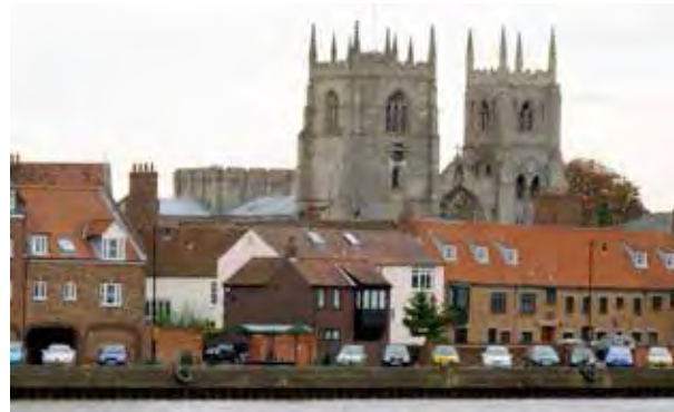
View of the St Margaret's area from the western bank of the river
