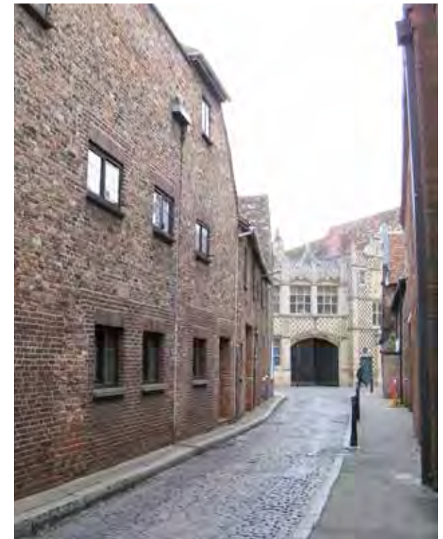
Historic paving in College Lane
