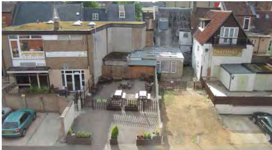
View of the back boundaries of Nos. 7-19 odd Tower Street from the first floor of the adjoining car park
