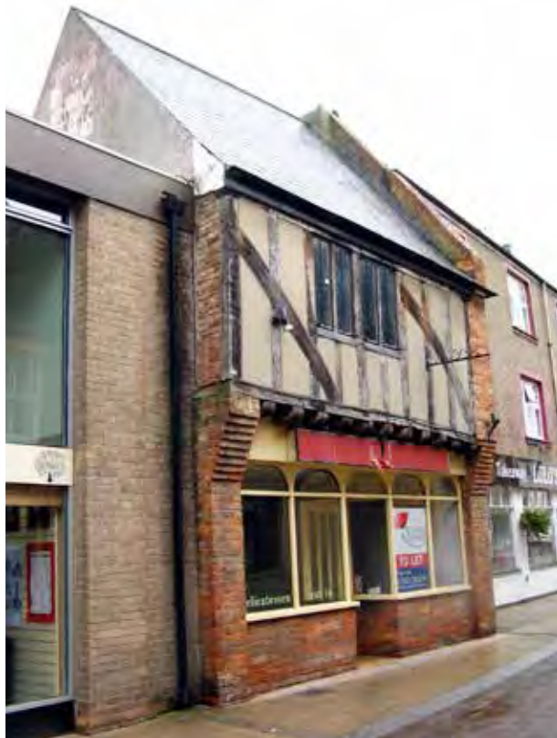
No. 21 Tower Street
