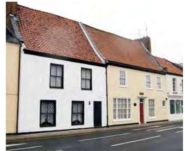
Nos. 17 and 18 Church Street
